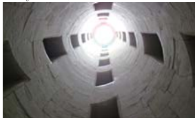
Captured from the base of the double-helix staircase designed by Leonardo da Vinci, located in the Chateau de Chambord in France. The staircase is counter-rotary, so that when two individuals take the stairs, their single hope to meet is never fulfilled, but the process itself is more than enigmatic and enjoyable.
